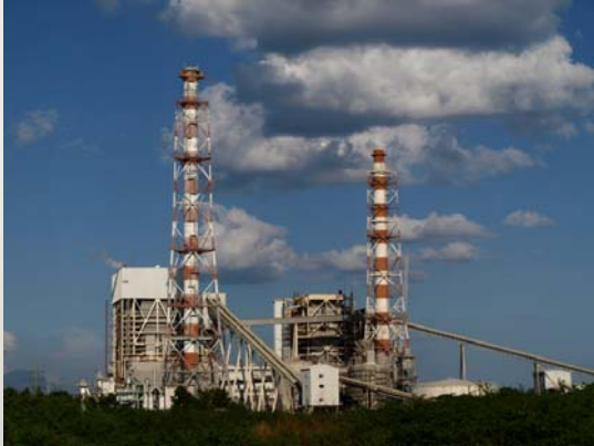
600 MW Batangas Coal-Fired Thermal Power Plant
